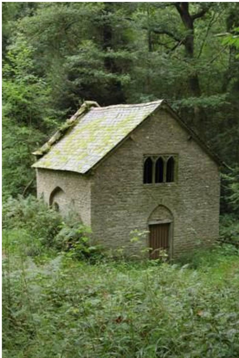
Inside the building Rex Wailes noted the presence of a beam which had notches, presumably for joists, showing that there had been, at one time, an intermediate floor and he was of the opinion that the pumphouse had originally been built as a corn mill and then, in the last quarter of the nineteenth century, gutted and converted into a water pumping mill. This major reconstruction was carried out by William T. Kevill-Davis (see *'History of Croft 1800-1923'*).
